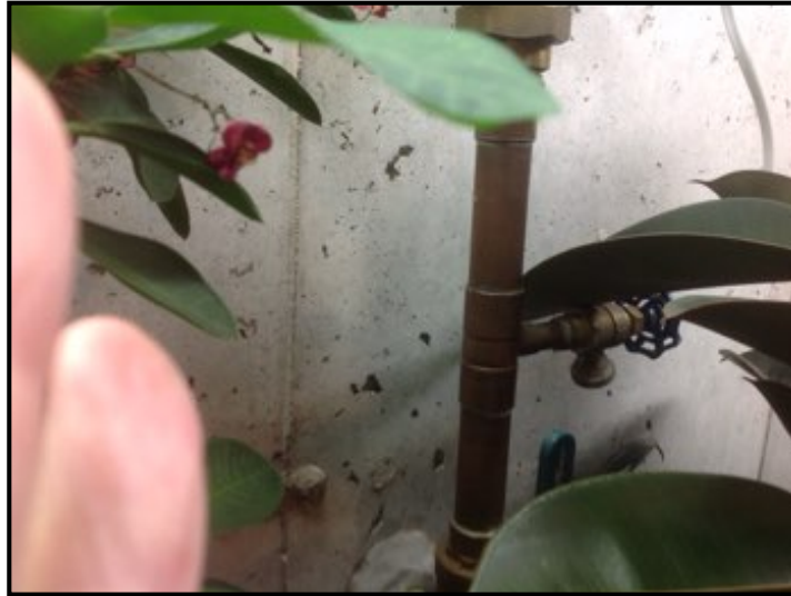
Water shutoff on east basement wall.
