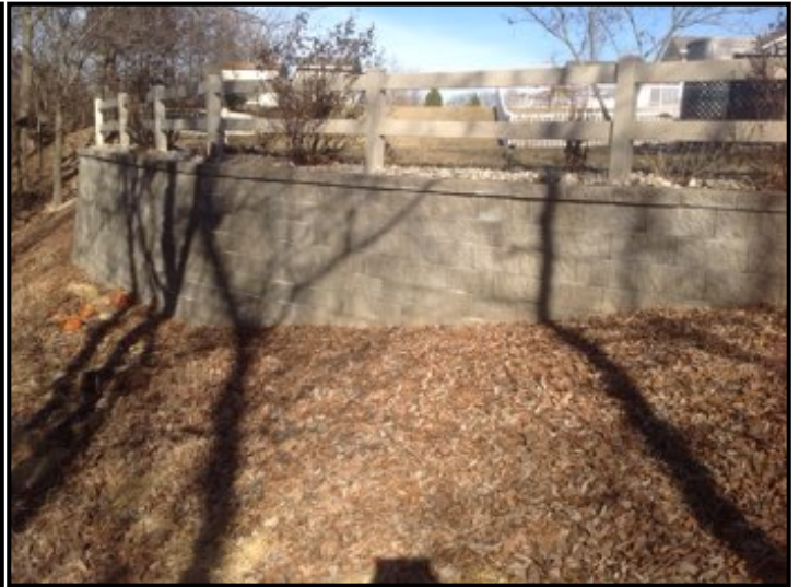
Retainer wall in good condition.
