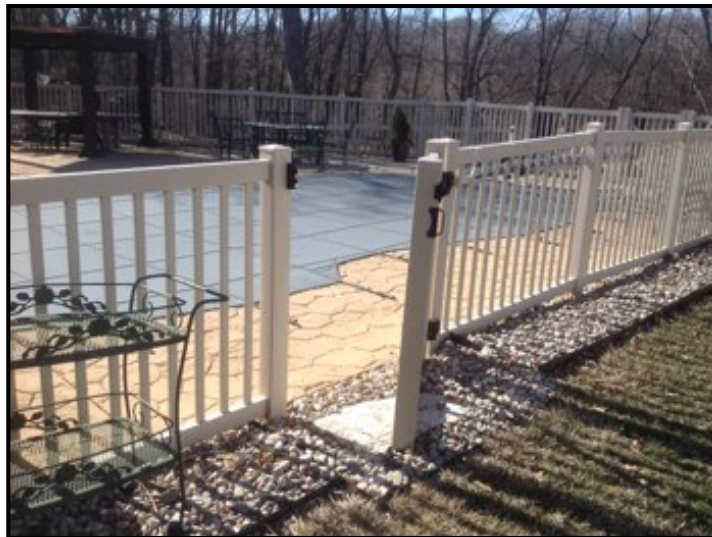
Gates require adjustment.
